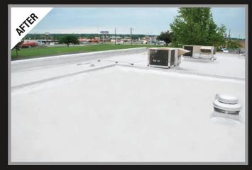
**PROBLEM:** Standing or ponding water on a roof can cause leaks and destruction. These damaging effects can be costly for the building owner. Acrylic roof coatings can't hold up to standing water. In the last few years, building owners have come to realize that ponding water resistance is a critical component in roof restoration coatings.
