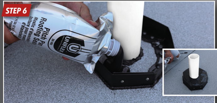
Use the Uniflex Pitch Pan Roofing Sealant to fill the Uniflex Pitch Pan Pocket cavity and tool as needed. Allow Uniflex Pitch Pan Roofing Sealant to fully cure. Tack Free: 40 minutes @ 75°F / 50% RH. Cure Time: Dependent about thickness: Approx 1/8" to 1/4" cure per week
