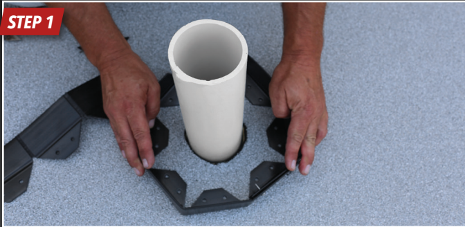
Size the fencing to fit the application. A two-inch gap between the fencing wall and penetration should be maintained.
