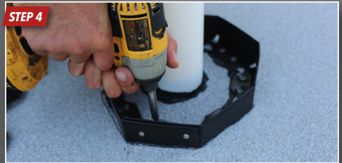
Position the UNIFLEX® Pitch Pan Pocket to the UNIFLEX® MS Hybrid Roofing Sealant outline and mechanically secure with mechanical fasteners.
