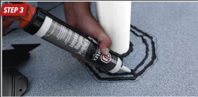
Place the UNIFLEX® Pitch Pan to the side, and seal around the perimeter of the penetration with UNIFLEX® MS Hybrid Roofing Sealant and over the traced pitch pan outline.
