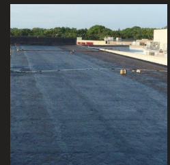
ASPHALT/BUR/ GRANULAR CAP SHEET
